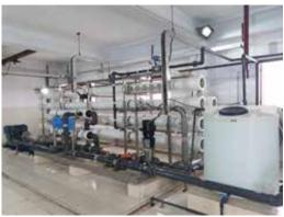
components, such as fresh water, while preventing passage of larger molecules, like salts and other impurities. The overall recovery of the water is about 62%. The water has been utilised in process, dying and utility purposes by the company.
